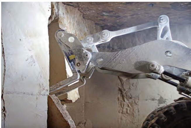
Tractor breaking out rubbish stone from face with forks
